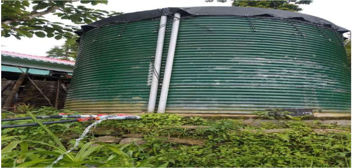
30,000ltrs Steel Demountable Water Harvesting Tank Name of Beneficiaries: Community Basis. Name of Land Donor :Phurba Lepcha Location: Paiyoungram
